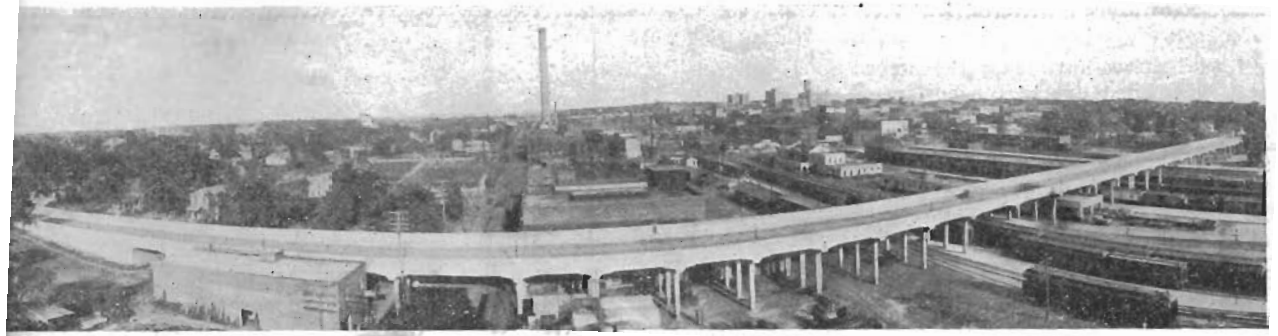
The Grant Avenue viaduct, across the Frisco's tracks on the north side of Springfield, Mo., and near the Frisco passenger station, was opened to traffic the night of September 11, immediately following a dedicatory celebration. The Frisco station is the Spanish mission style building a little to the left of the center of the picture.
