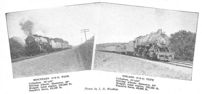
N the Spring of 1923, the St. Louis-San Francisco Railway placed in operation fifty Baldwin locomotives—fifteen of the Mountain (4-8-2) type and thirty-five of the Mikado (2-8-2) type, designed to make long runs and handle heavy tonnage under difficult operation conditions.
