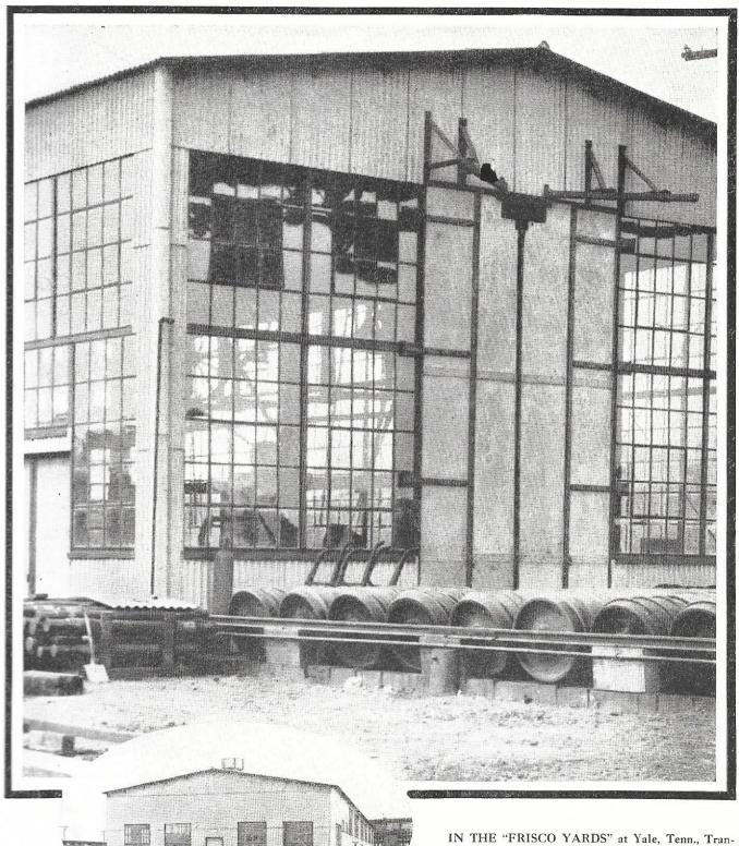
IN THE "FRISCO YARDS" at Yale, Tenn., Transite is used for roofing and siding on the car wheel shop, machine shop, car department, power house and other buildings. Ventilators, interior partitions, the smoke jacks in the roundhouse, even the enormous doors of the car wheel shop (shown above) are made of this durable material.
