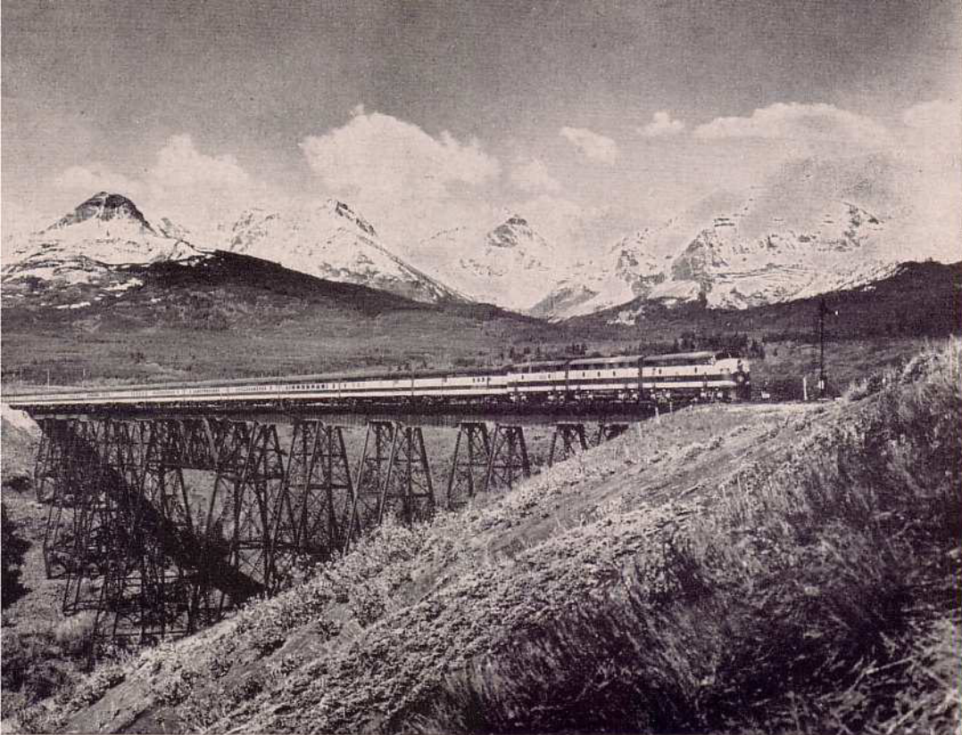
SPANNING STREAM AND VALLEY
